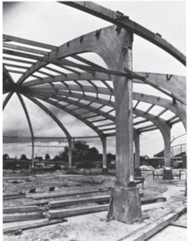
FIGURE 19.1.3 A Variation of Type IV (Heavy Timber) Construction with Haunched Arches of Laminated Wood (Glue-Laminated Construction) and Beams Anchored to Arches by Steel Hangers
