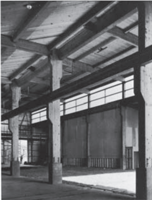
FIGURE 19.1.2 Elements of a Building of Type IV (Heavy Timber) Construction. Note the large size of the columns and beams and the absence of concealed spaces. The exterior nonbearing wall at far left is of lightweight corrugated steel.
